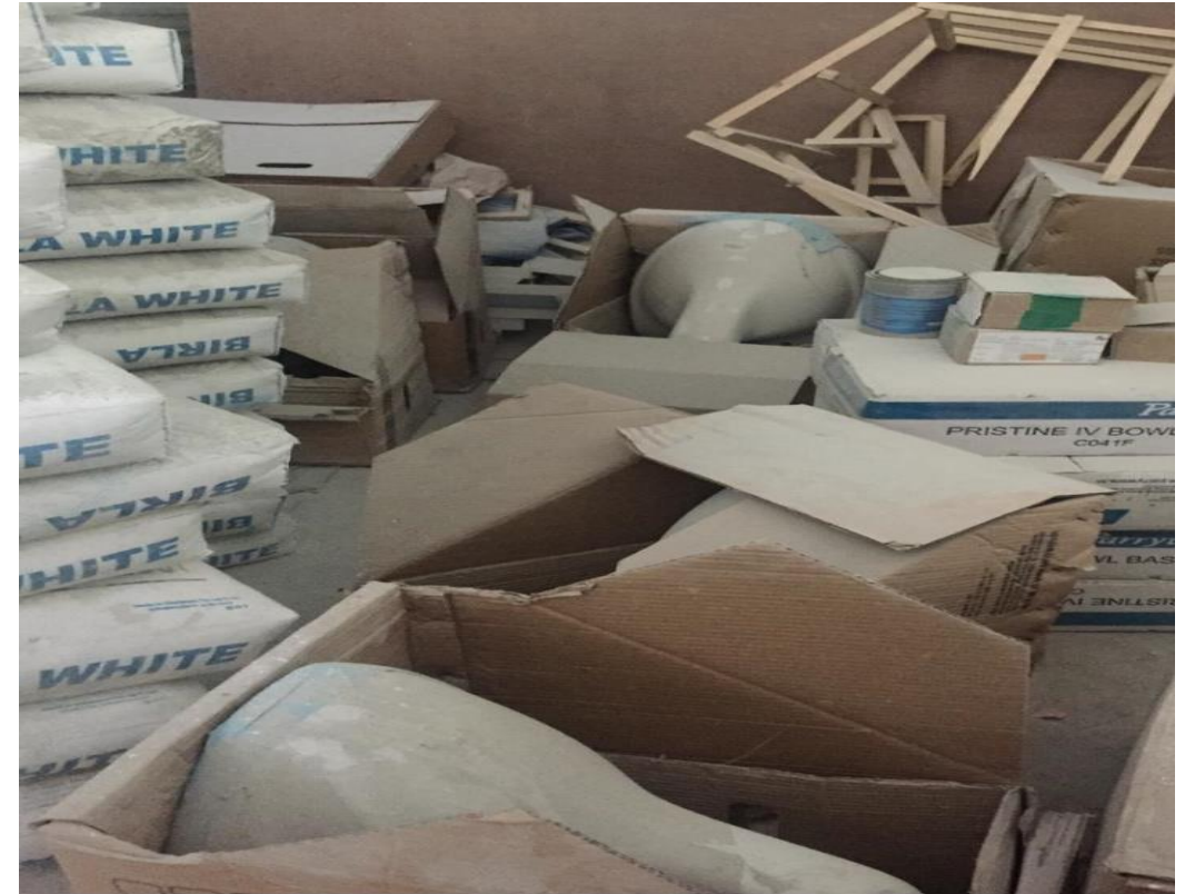
2. Box of materials are kept open after the seal is broken
